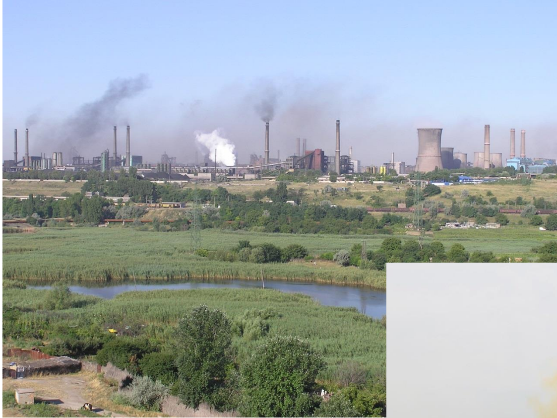
Galati Arcelor Mittal Steel factory
